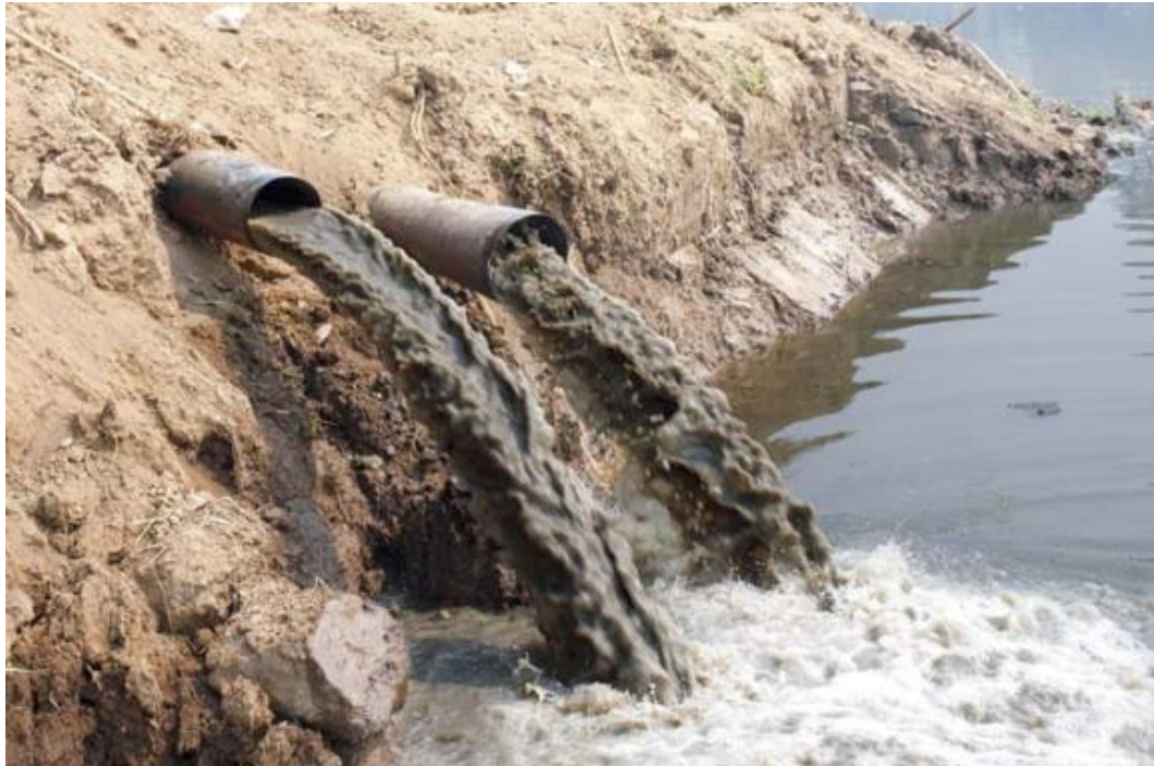
Fig 3: A typical storm water outfall, subject to water quality law
