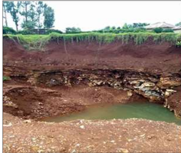
D. Water Infiltration through Slope Face
