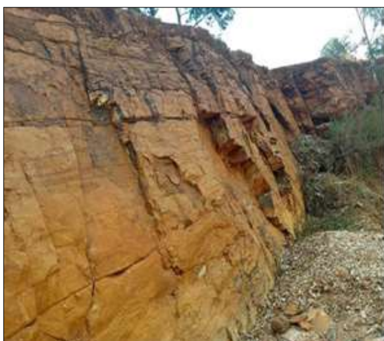
A. Rock Discontinuities (joints, cracks)
