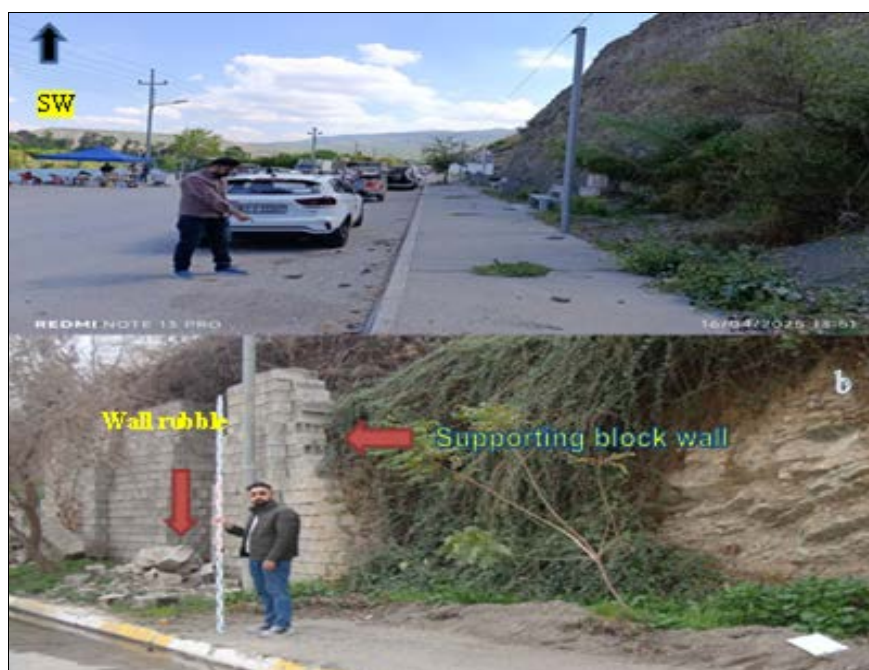
Fig 3a: Station 4: Side view of a rock fall on Middle Street, (Fig 3b) Station 1: Side view of a wall and debris material Using (Leveling Rod), Fig (3a) demonstrates the rock fall incident at Station 4, with rock fragments descending the slope, surpassing the curb, and reaching
