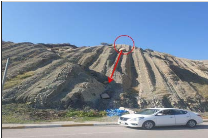
Fig 4: Station 4 on the slope showing the collapse of large rock masses down the slope due to weathering, erosion, and gravity.
