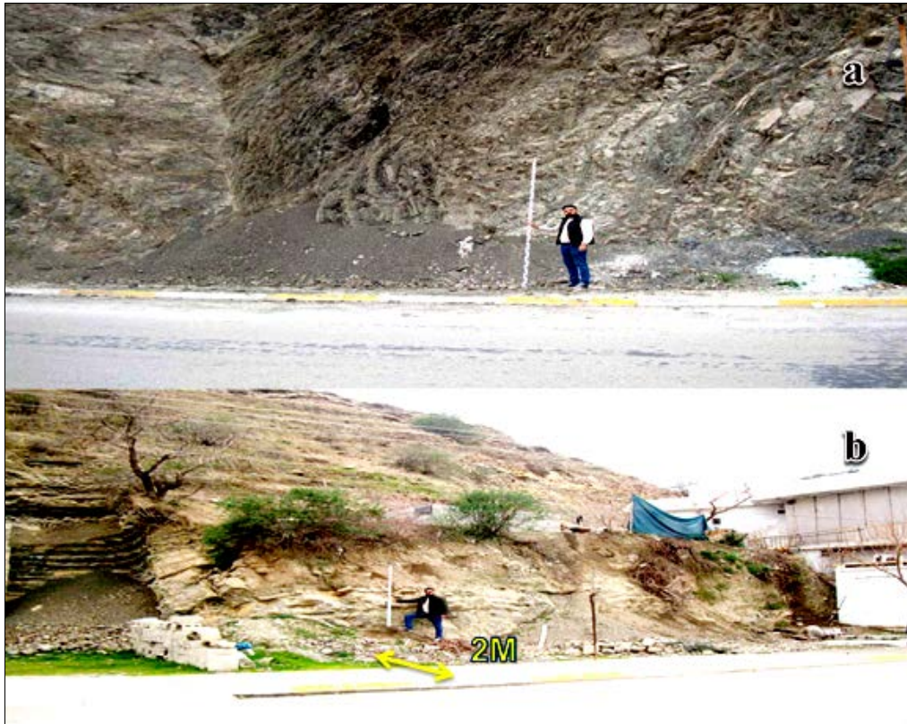
Fig 5a: Station No.2 The photo is taken in the direction of 072°, showing the slope face. However, the entire height of the slope could not be captured by the camera. (Fig.5b) It shows that the sidewalk is narrow, with a width of approximately 2 meters.
